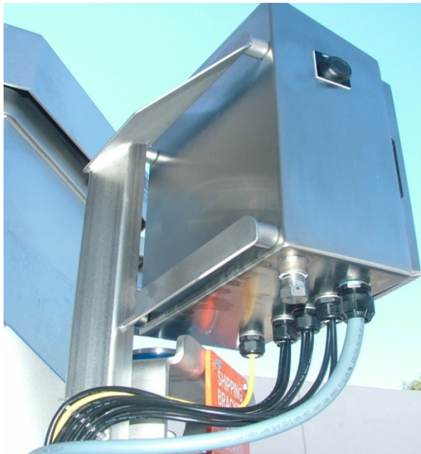
<<Cable Enters Bottom of Panel
