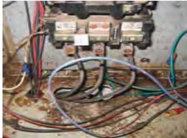
Corrosion leads to premature component failure
