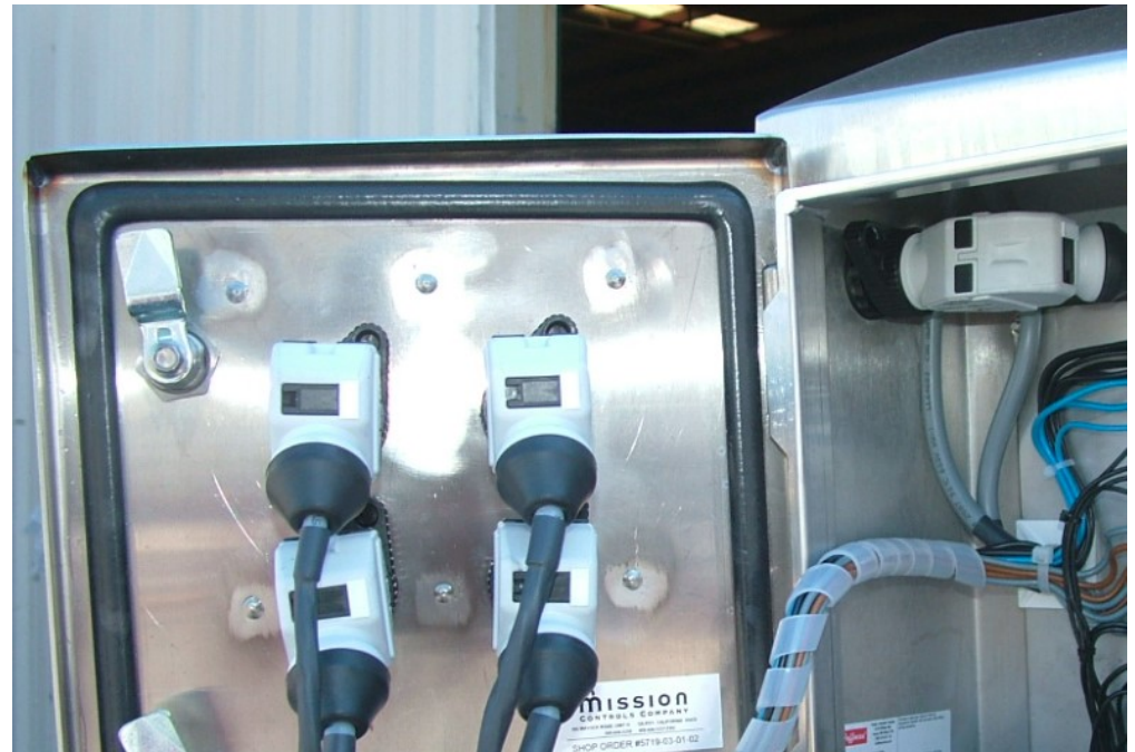
Hermetically sealed push buttons
